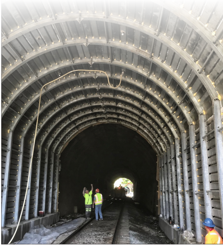
Installation of arch sets and backfilling in railroad tunnel.
